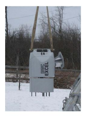
6. Use the crane to lift the powerhead, still attached to the shipping skid, clear of the ground using a double-eye nylon strap. Slip one eye over each end of the tail pivot pin and onto the mainframe; hook the crane line to the center of the strap and lift. The shipping nuts can now be removed from the blade studs so the skid can be pulled off and set aside.
