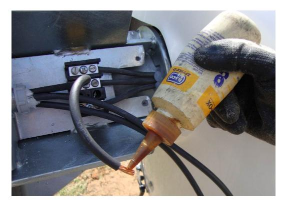
e. Trim each of the conductors to a length that will allow formation of full 360° strain relief loops to each terminal connection. Strip each of the three conductor wires back 3/4" (2 cm), apply anti-oxidation compound to the bare copper and make connections to the terminal block. All three wires are equivalent; there is no polarity or required phase rotation.
